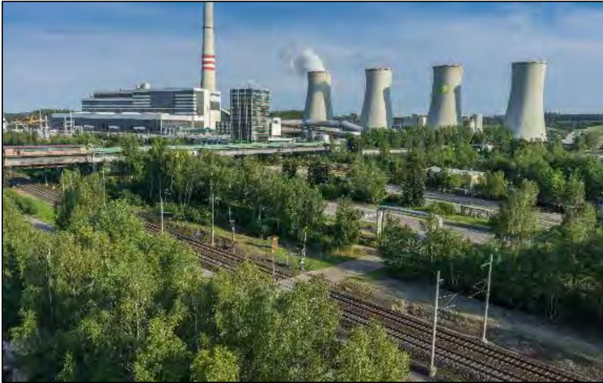
Figure 6-3: Current Power Plant
