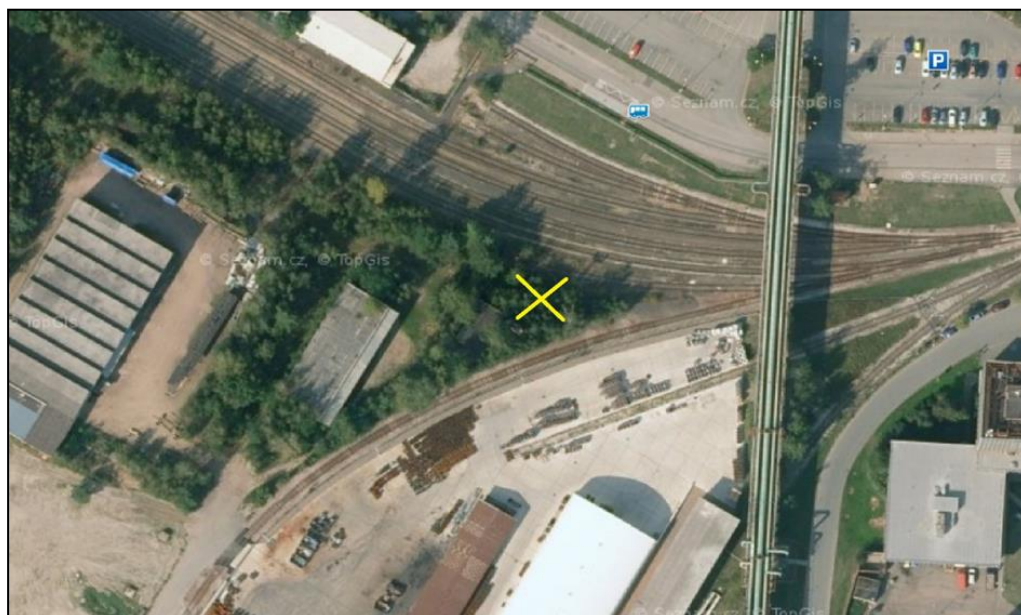
Picture no. 41: Approximate position of 400kV cable input to the processing plant area
