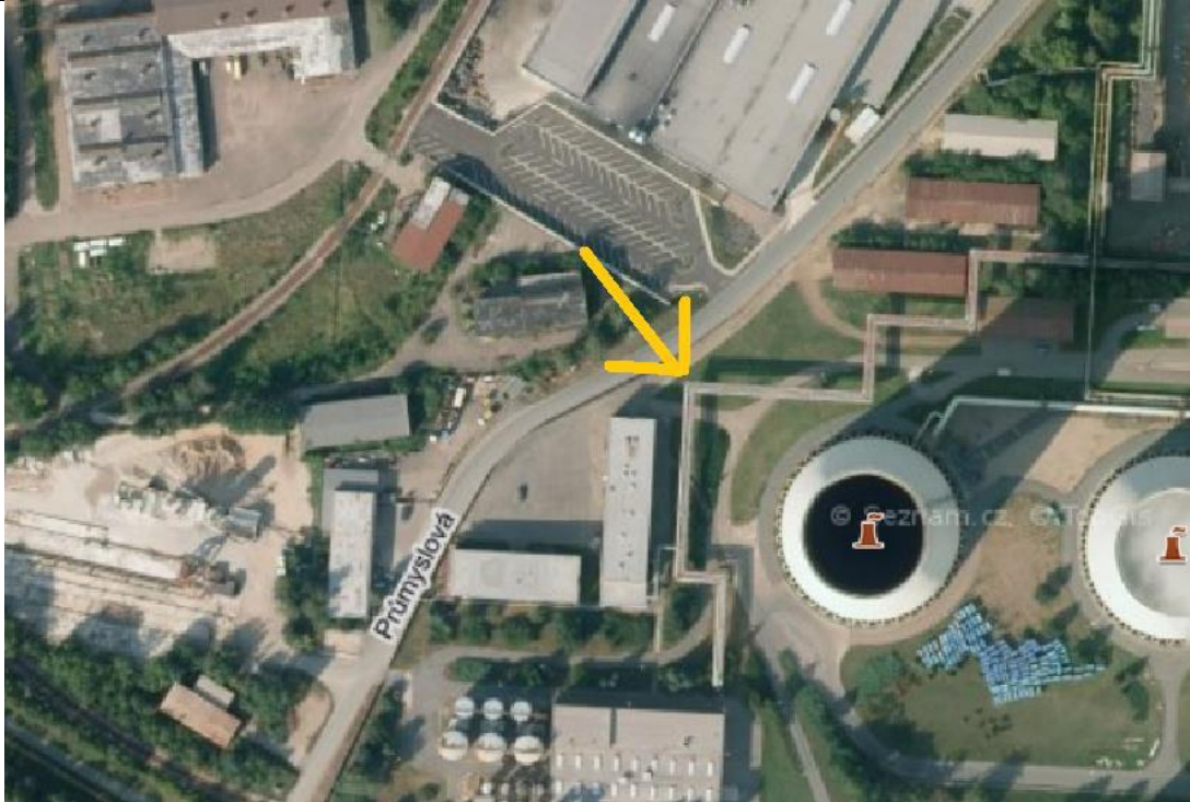
Figure 7: Connection point for superheated water from the Chvaletice Power Plant
